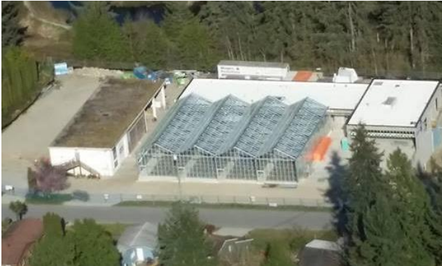
SECHELT BC – Wastewater Treatment Plant, ADWF Capacity 2.0 MLD existing, 4.0 MLD future
