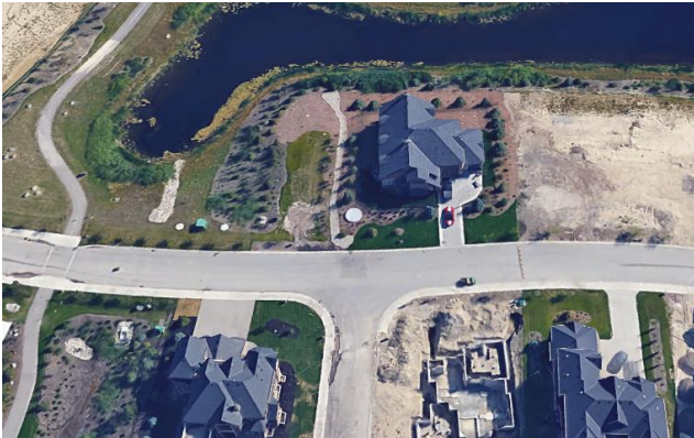
ROCKY VIEW COUNTY AB – Watermark at Bearspaw WWTP, Capacity 0.7 MLD existing
