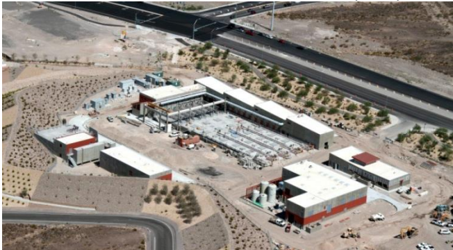
HERDERSON NV - Southwest WRF, AAF Capacity 30 MLD existing; expandable to 60 MLD
