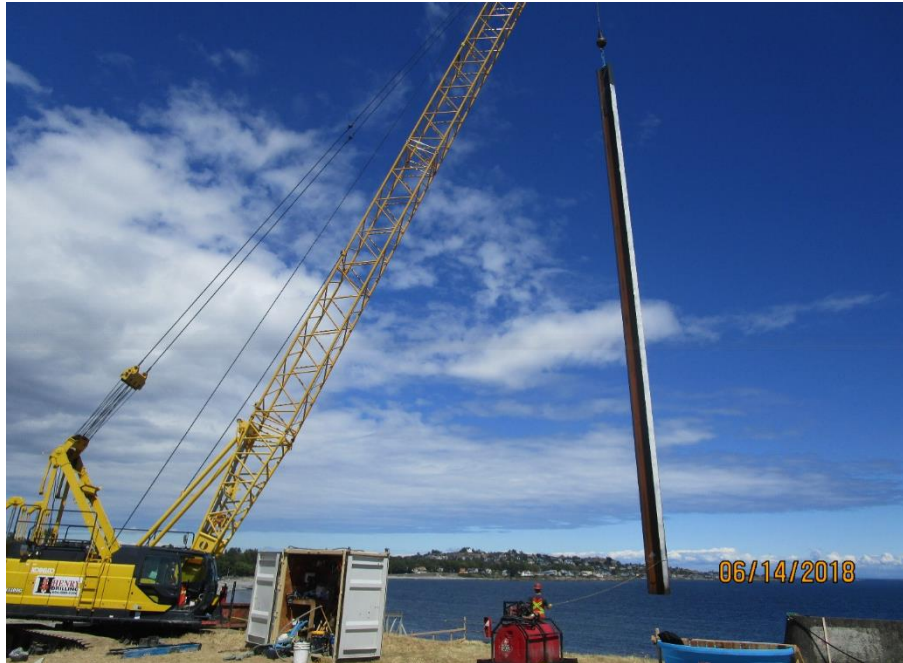
Figure 12 – Hoisting king pile #17 into place.
