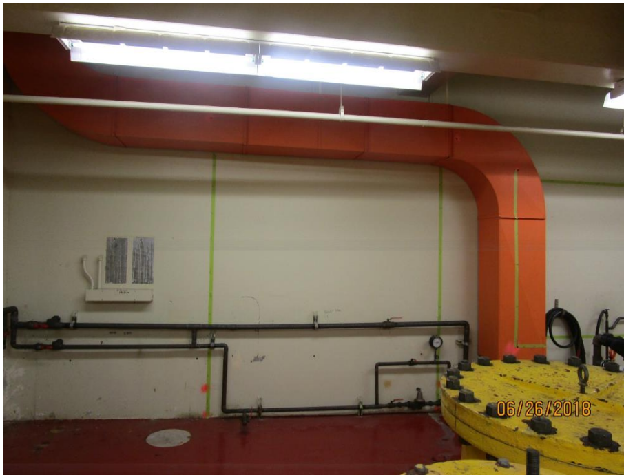
Figure 13 – Layout of future opening for new corridor and outfall pipe path at lower level.
