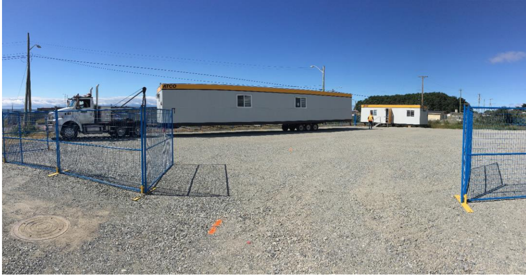
Figure 14 – Kenaidan second office trailer delivered to site
