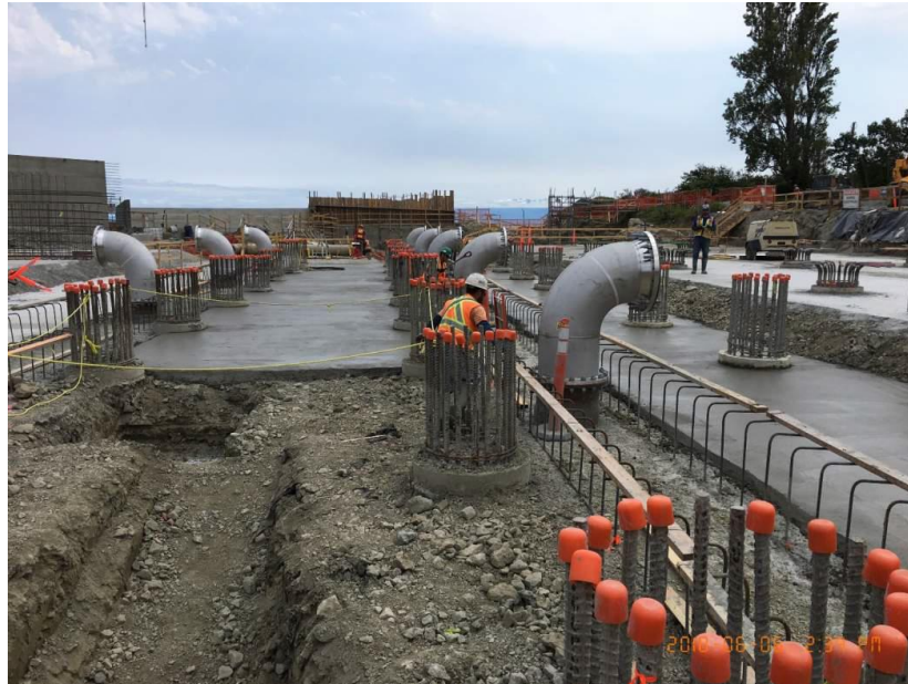
Figure 5 – Mudslab placed in central biological aerated filters (BAF) area.
