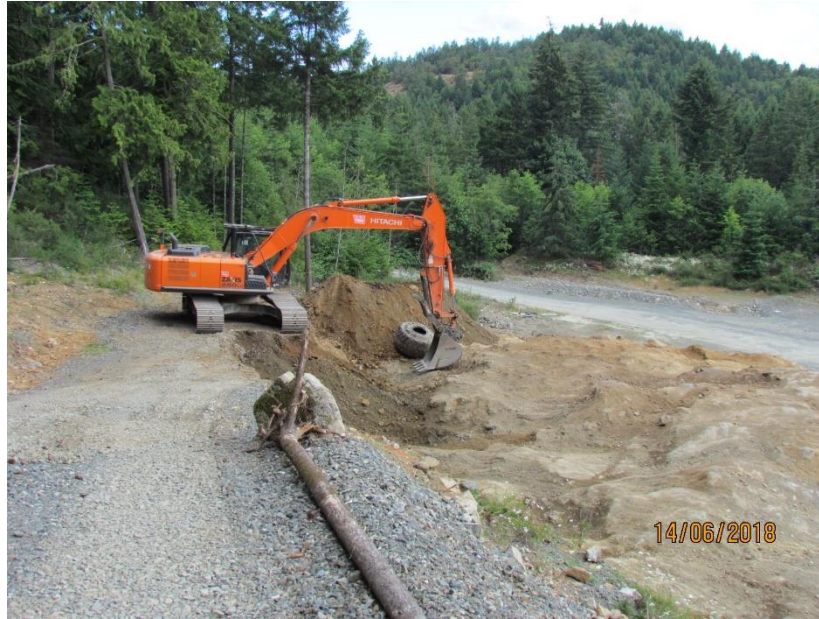
Figure 9 – Stripping of organics from blast area.
