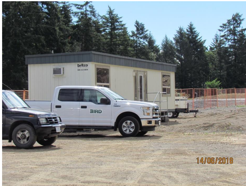
Figure 10 – Office trailer with temporary power connected.
