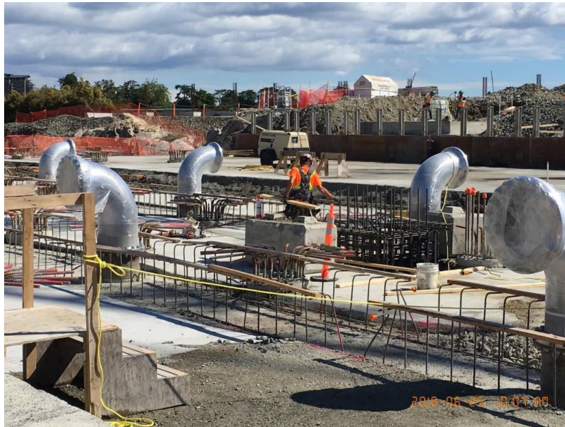
Figure 8 – Setting rebar cages for biological aerated filters (BAF) gallery sumps.
