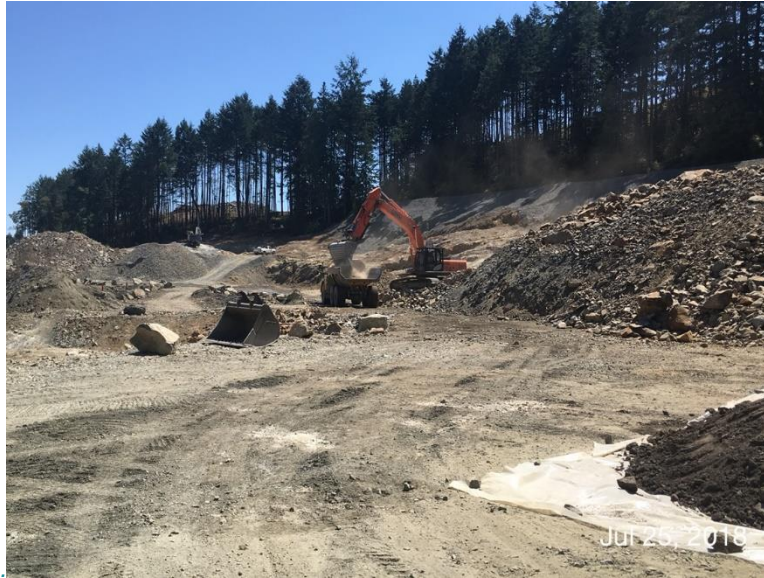
Figure 11 – Excavating and loading blast rock.
