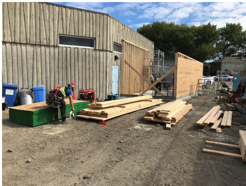
Figure 20 – Commence framing of temporary bin room.
