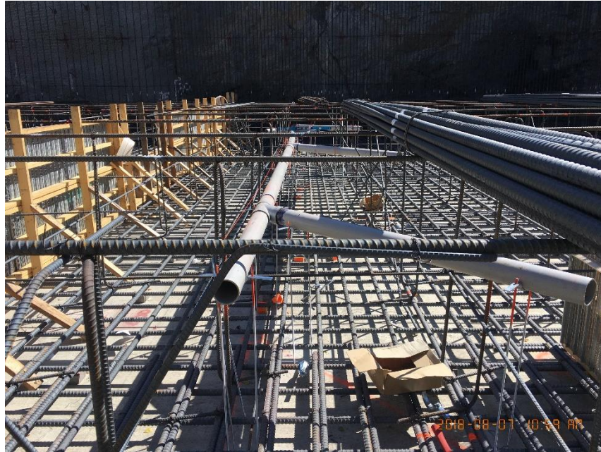
Figure 4 – Setting floor drains in the tertiary slab.
