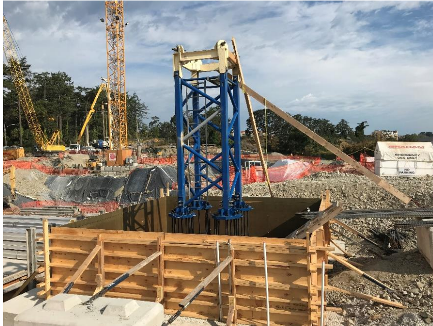
Figure 2 – Preparing foundation for concrete placing boom.
