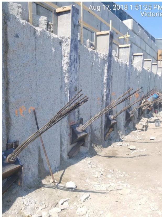
Figure 17 – Tension and proof testing tie-backs.
