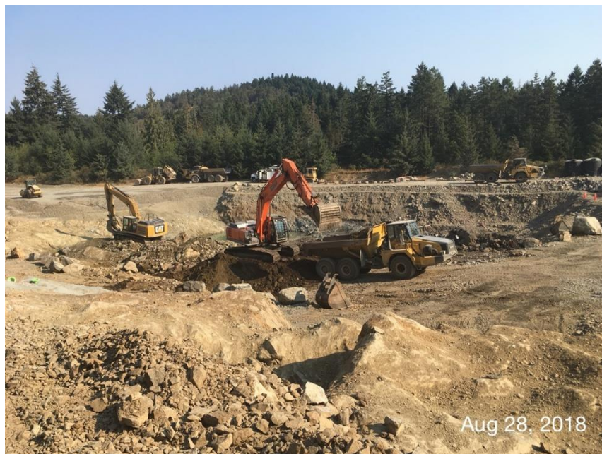
Figure 12 – Loading and hauling contaminated material to Hartland Landfill.
