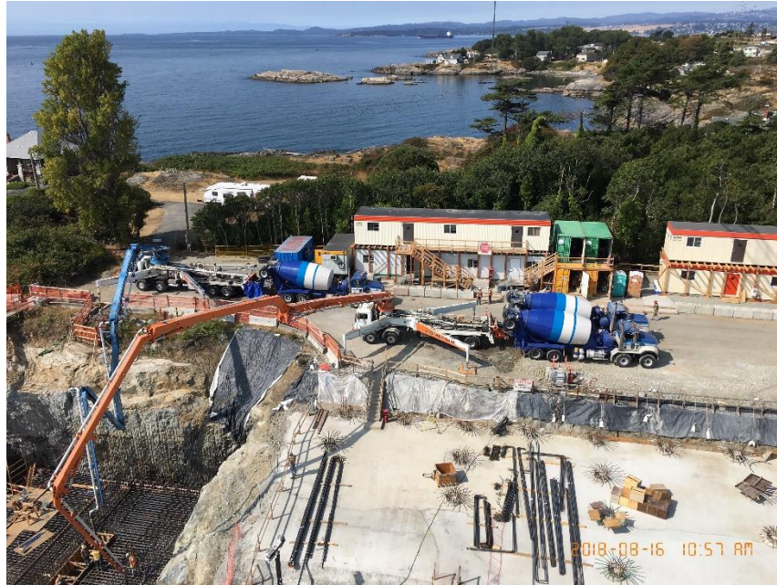
Figure 6 – Placing concrete in the tertiary slab.
