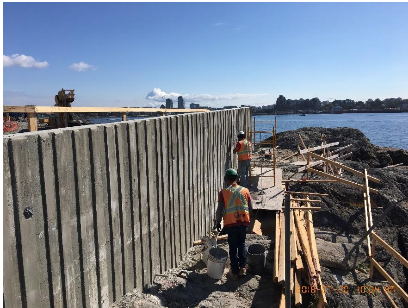
Figure 6 – Concrete finishing of planter wall #10.
