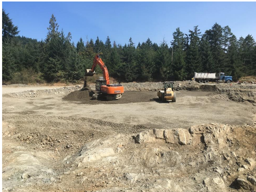
Figure 10 – Spreading and compacting aggregate at digester #1 location.
