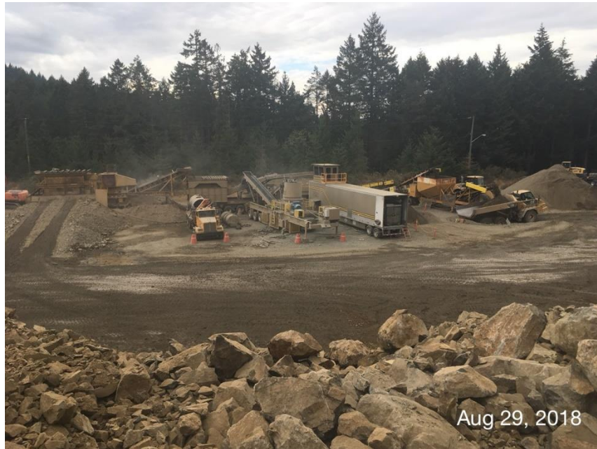
Figure 9 – Rock crushing plant in operation.
