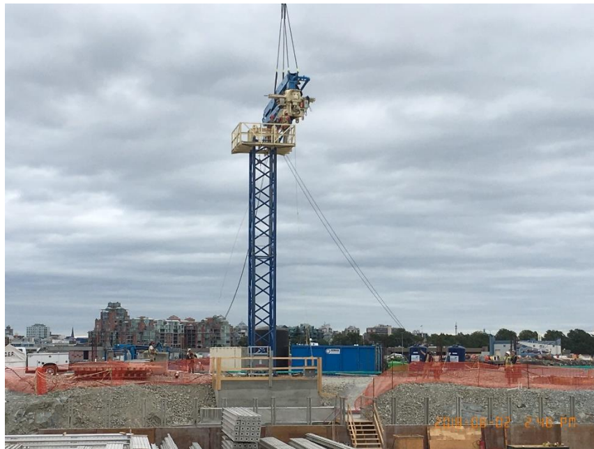
Figure 3- Erecting concrete placing boom for operations and maintenance (O&M) area.
