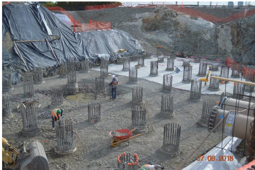
Figure 3- Preparing dirty back wash area for mud slab.
