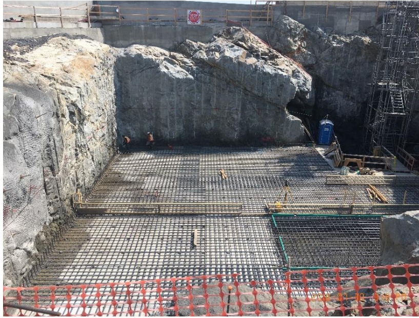
Figure 8 – Installing bulkheads in tertiary slab pour.
