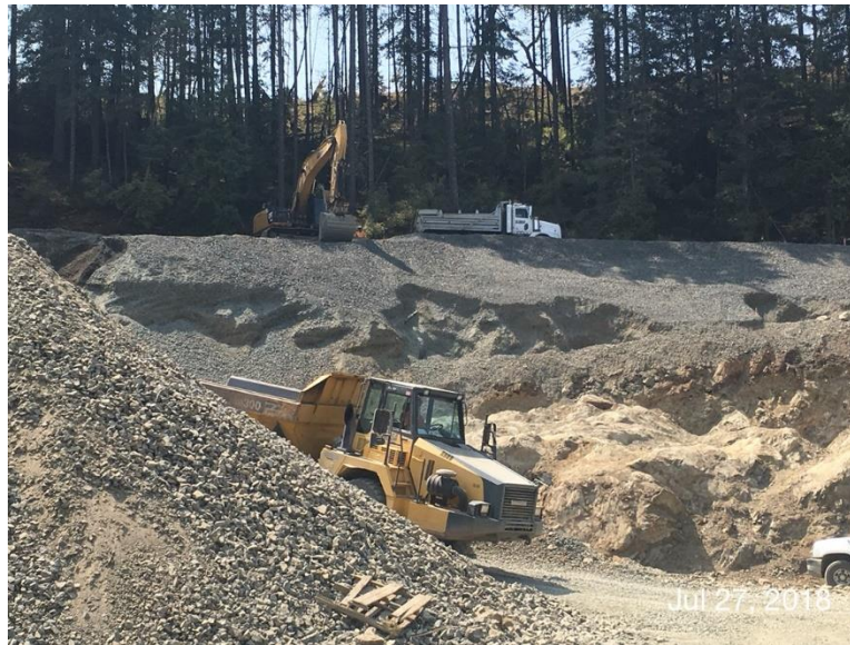
Figure 12 – Stripping and hauling at upper Hartland access road.
