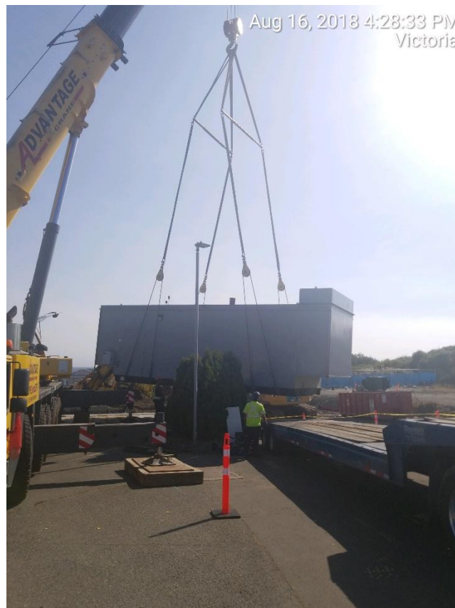
Figure 18 – Hoisting E-house and moving to new location.
