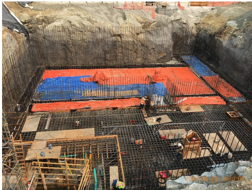
Figure 7 – Wet curing of concrete slab.
