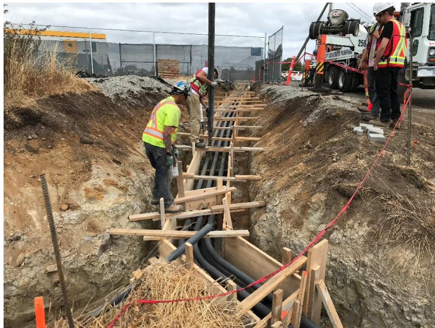
Figure 19 – Placing concrete in duct bank under View Point Road.
