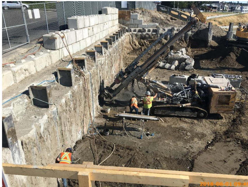
Figure 13 – Southwest drilling tie-backs.
