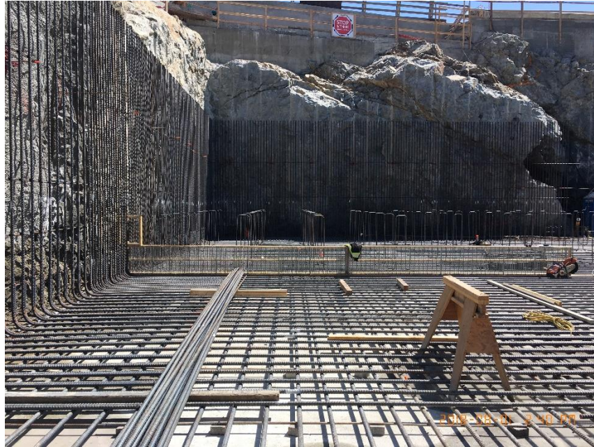
Figure 2 – Rebar dowels in the tertiary area.
