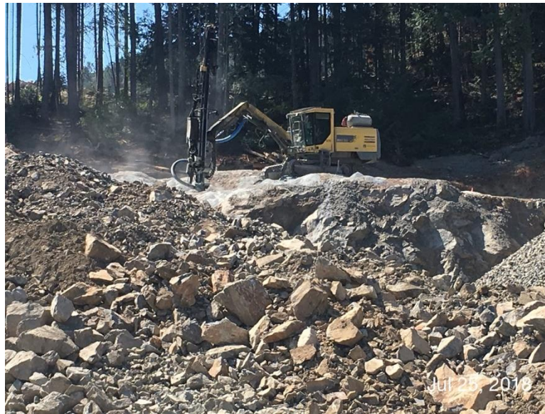
Figure 10 – Drilling holes for a blast
