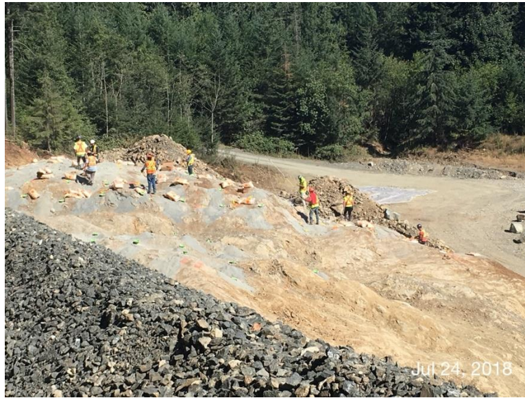
Figure 9 – Loading drill holes for a blast.
