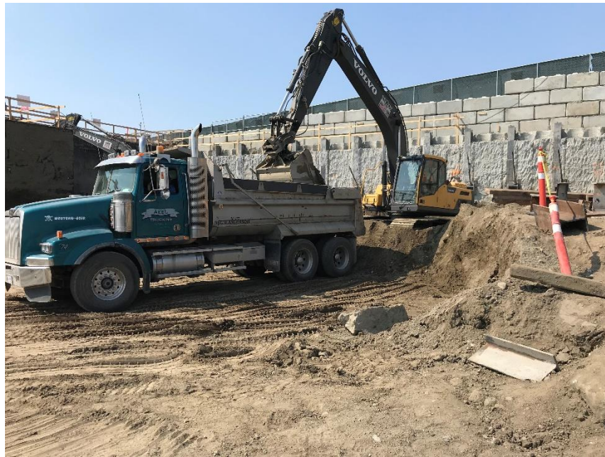
Figure 16 – Excavating down to lower level of tie-backs and hauling material offsite.
