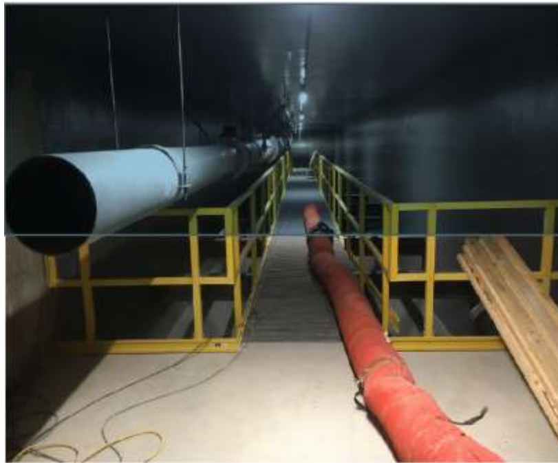
Figure 12-Macaulay Point Pump Station- Wet well fiberglass reinforced plastic platform installation.
