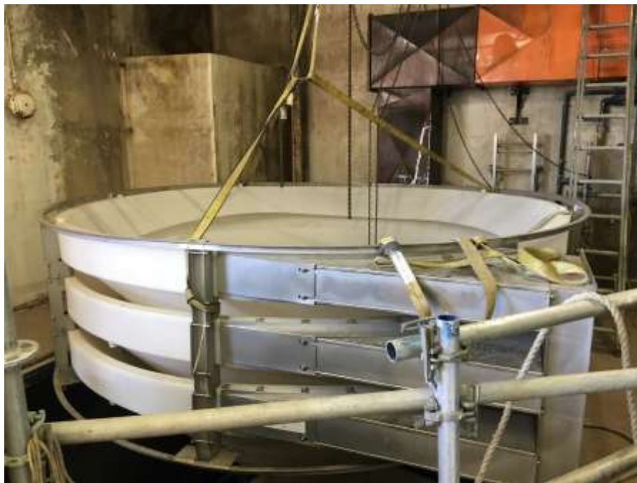
Figure 9–Clover Point Pump Station- Headcell installation.
