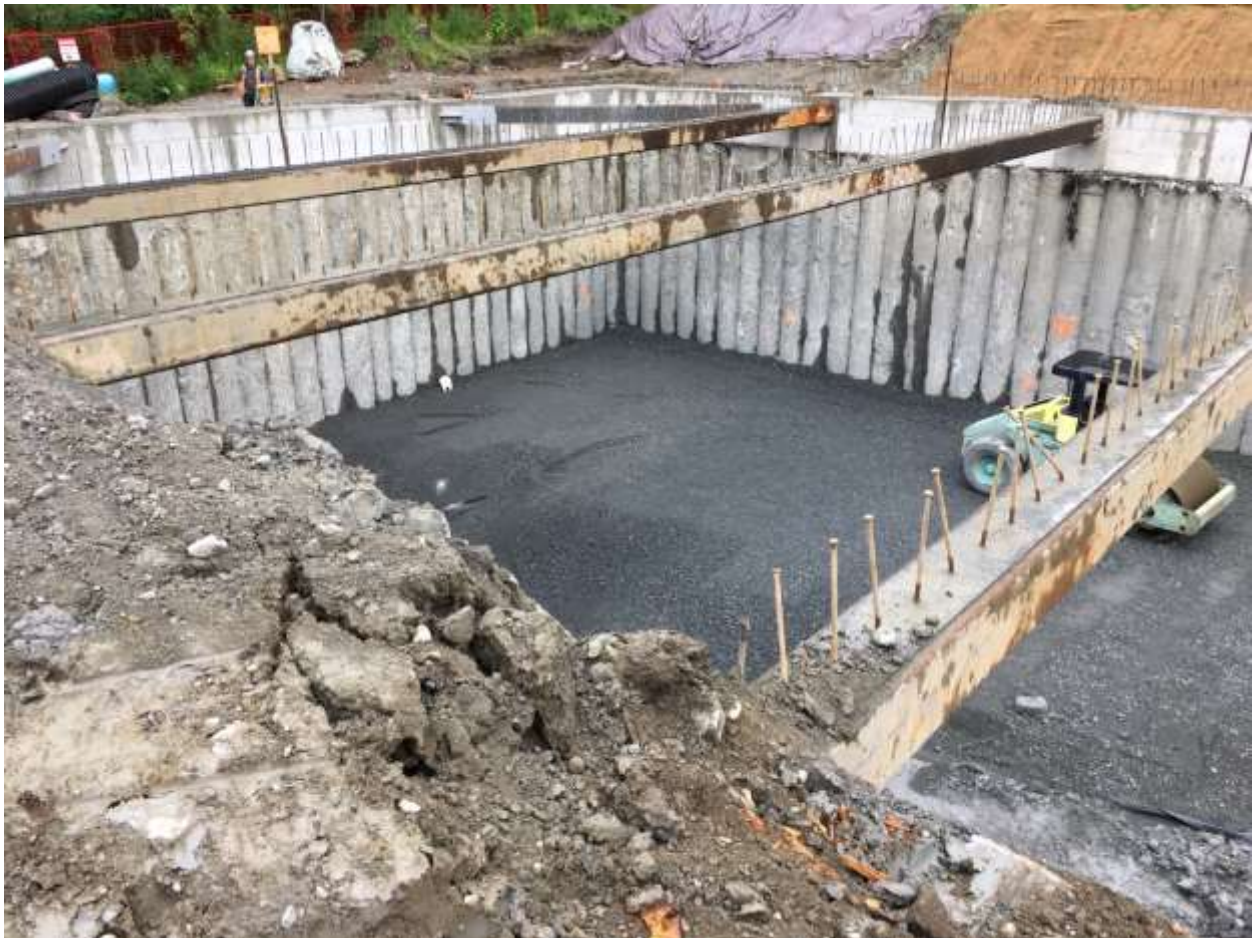
Figure 21–Arbutus Attenuation Tank- Excavation continues with placement of base course gravel installed.
