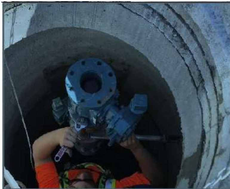
Figure 18-Residual Solids Pipes -Installing plug valves at Selkirk Ave.
