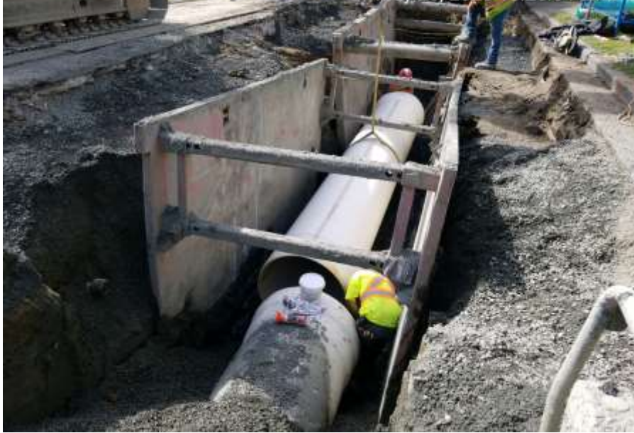
Figure 22- Trent Forcemain – Stannard Avenue – Forcemain installation progresses.
