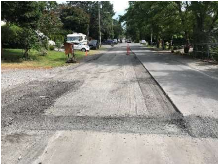
Figure 16– Residual Solids Pipes- Milling asphalt prior to paving on Grange Road.
