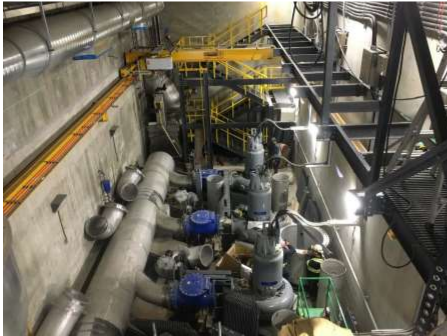
Figure 13-Macaulay Point Pump Station- Pump Room progression.
