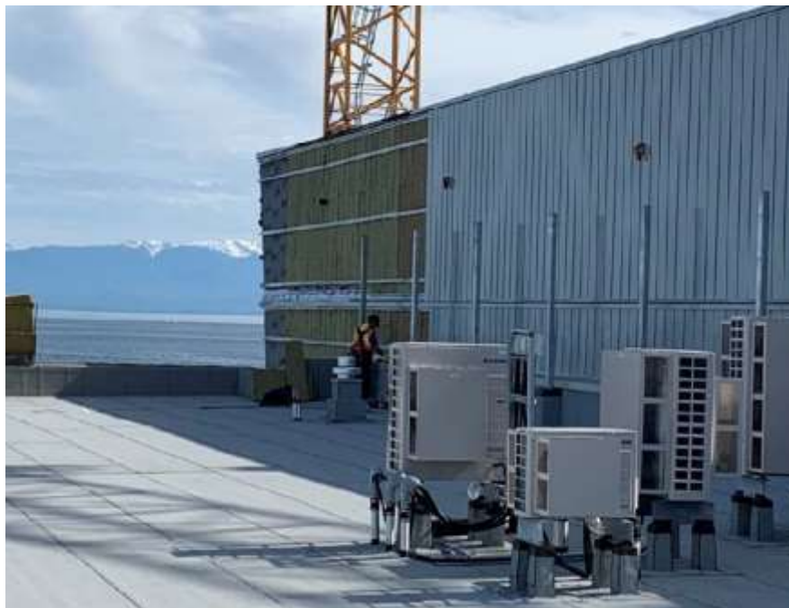
Figure 5- McLoughlin Point Wastewater Treatment Plant- Installing insulation and cladding on east face of Blower Building.
