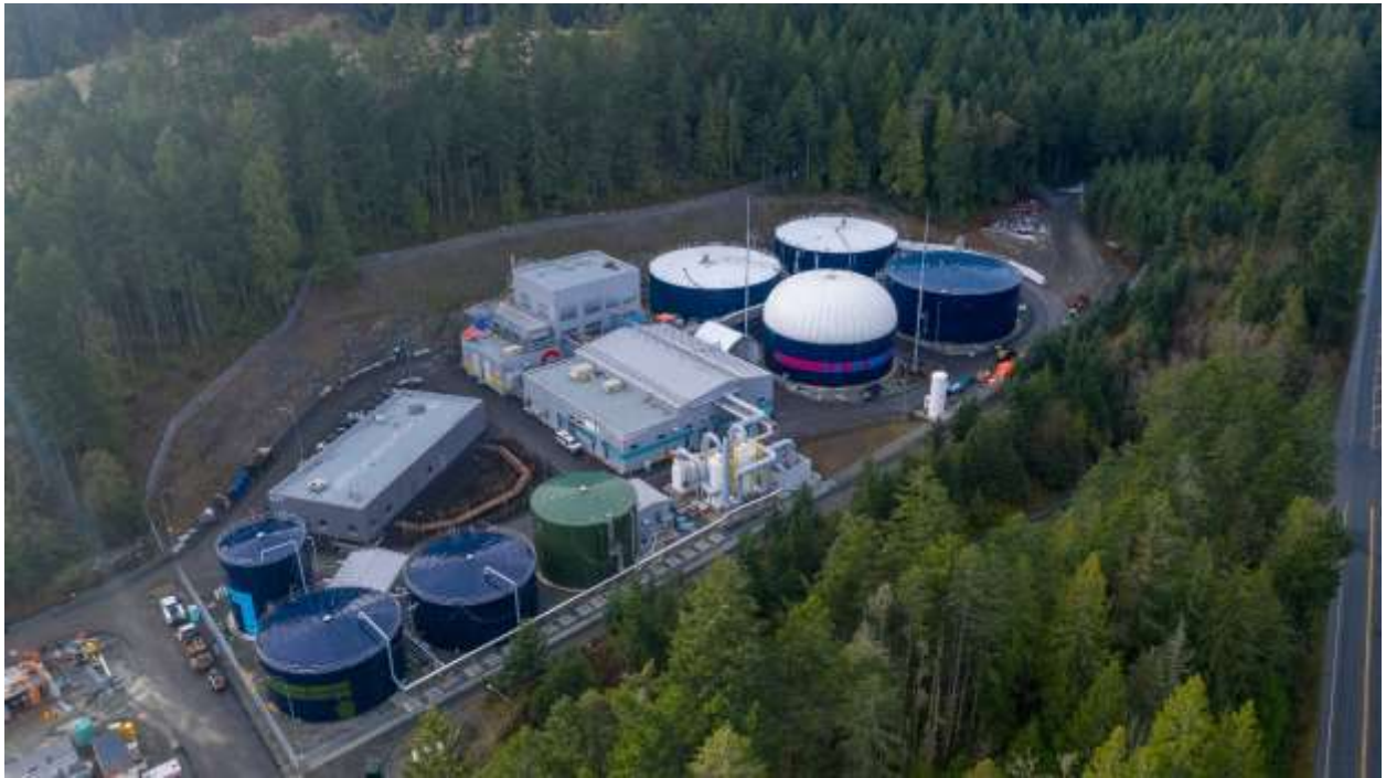
Figure 3 – Looking southwest toward the Residuals Treatment Facility
