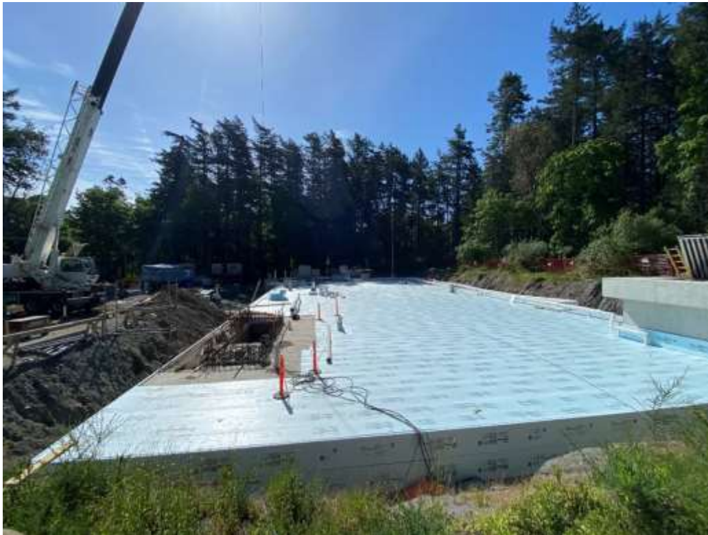
Figure 14 – Arbutus Attenuation Tank (Construction in progress)
