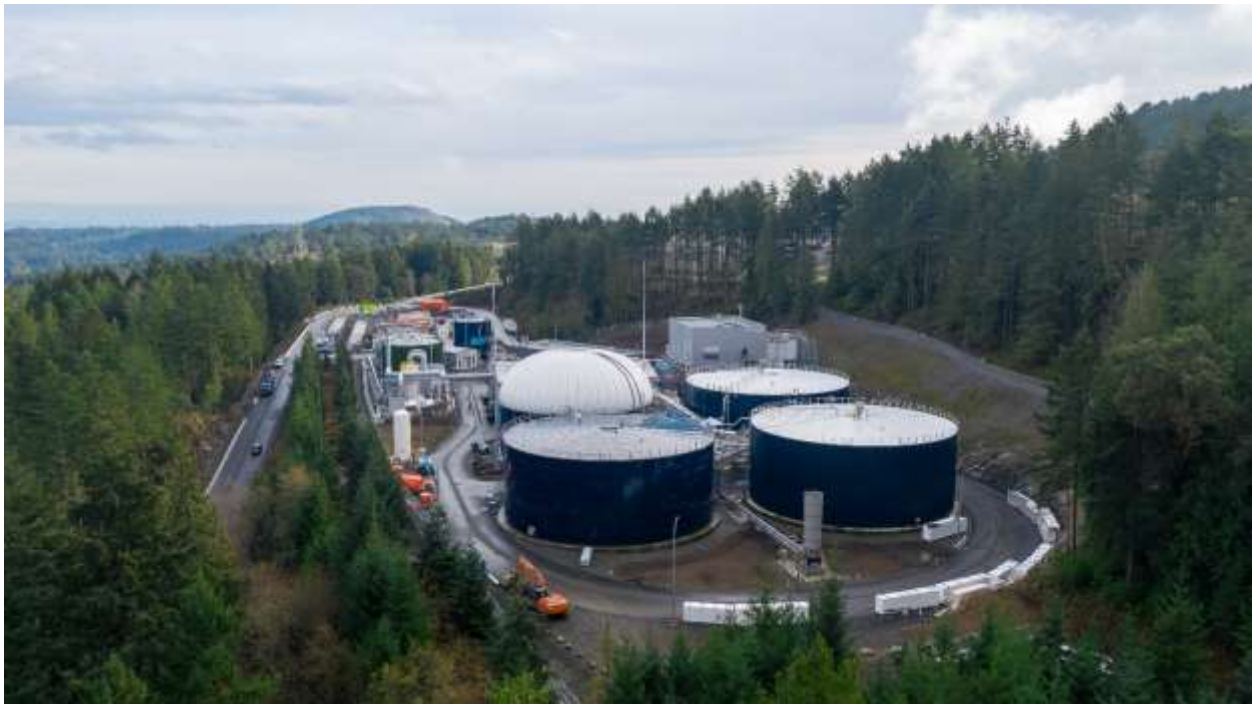
Figure 4 – Looking east toward the Residuals Treatment Facility
