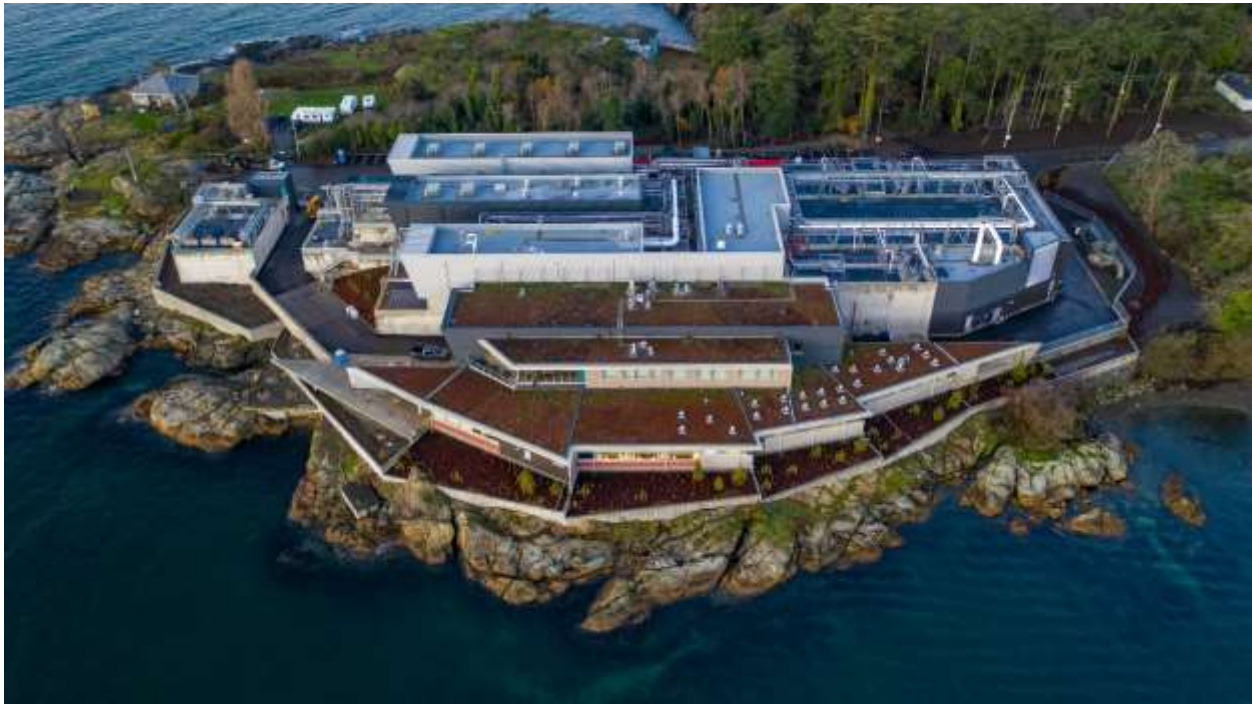
Figure 1 – Looking west at the McLoughlin Point Wastewater Treatment Plant
