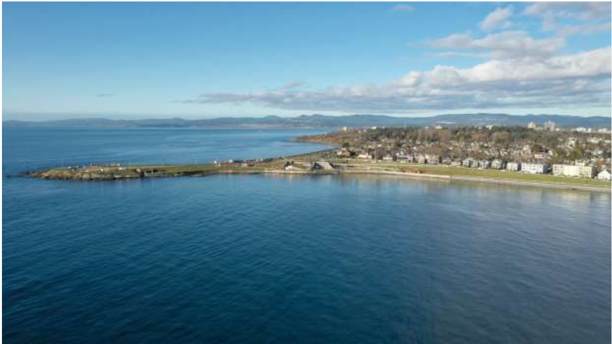
Figure 5 – Looking west towards Clover Point Pump Station (construction in progress)
