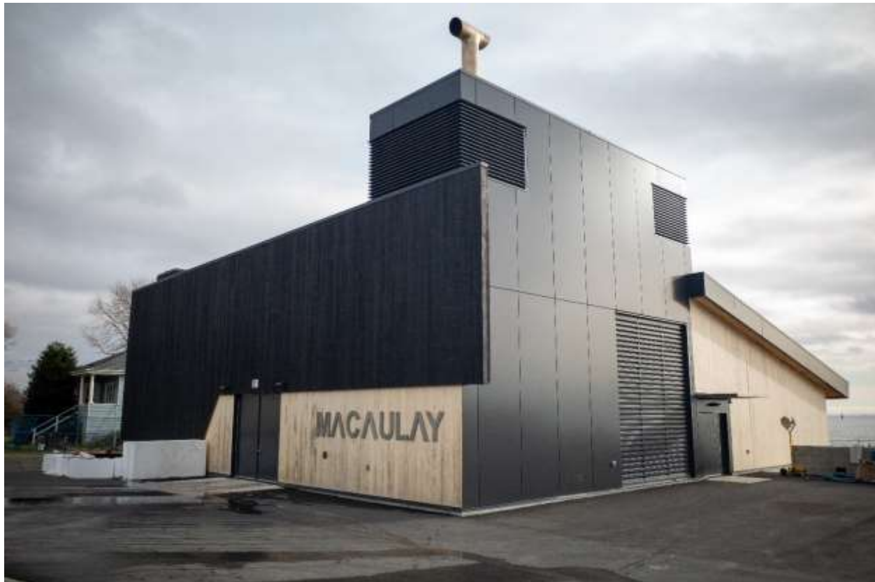
Figure 9 – Macaulay Point Pump Station
