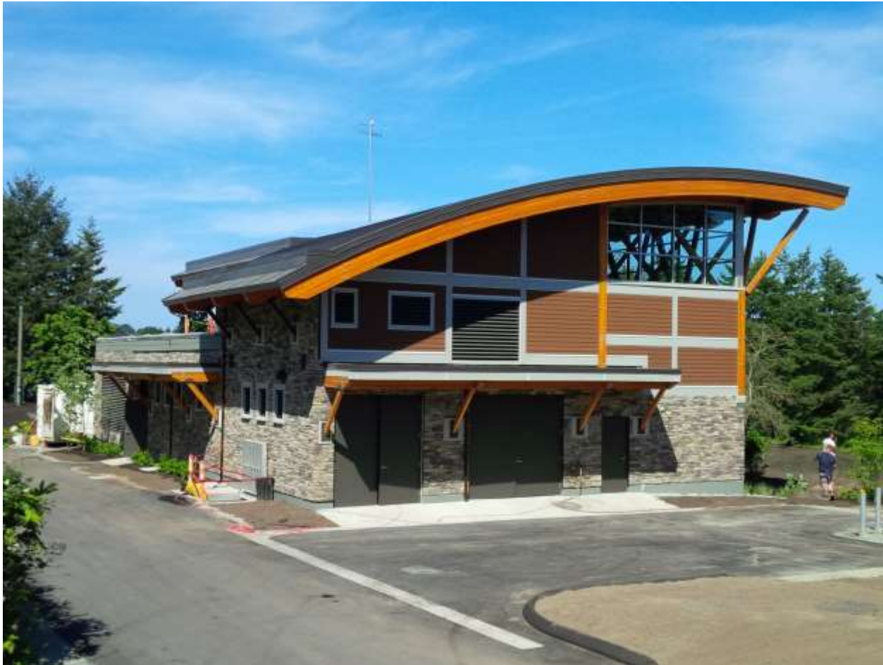
Figure 11 – Craigflower Pump Station
