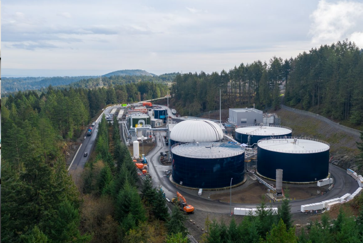
Residual Treatment Facility
