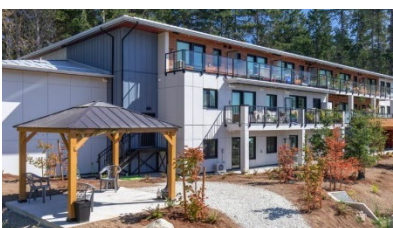
132 Corbett Rd. Phase III Opened 2022
