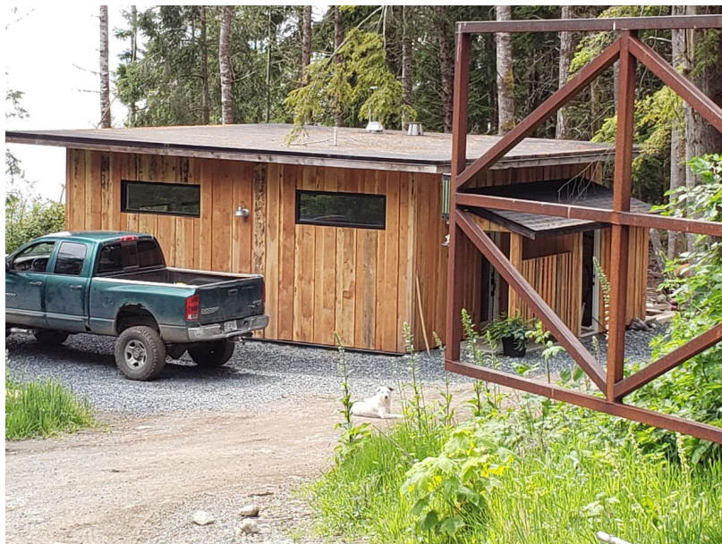
Detached Suite (work continued)
