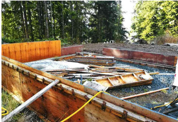
Secondary Building (footings and walls under construction without permits or approvals)
