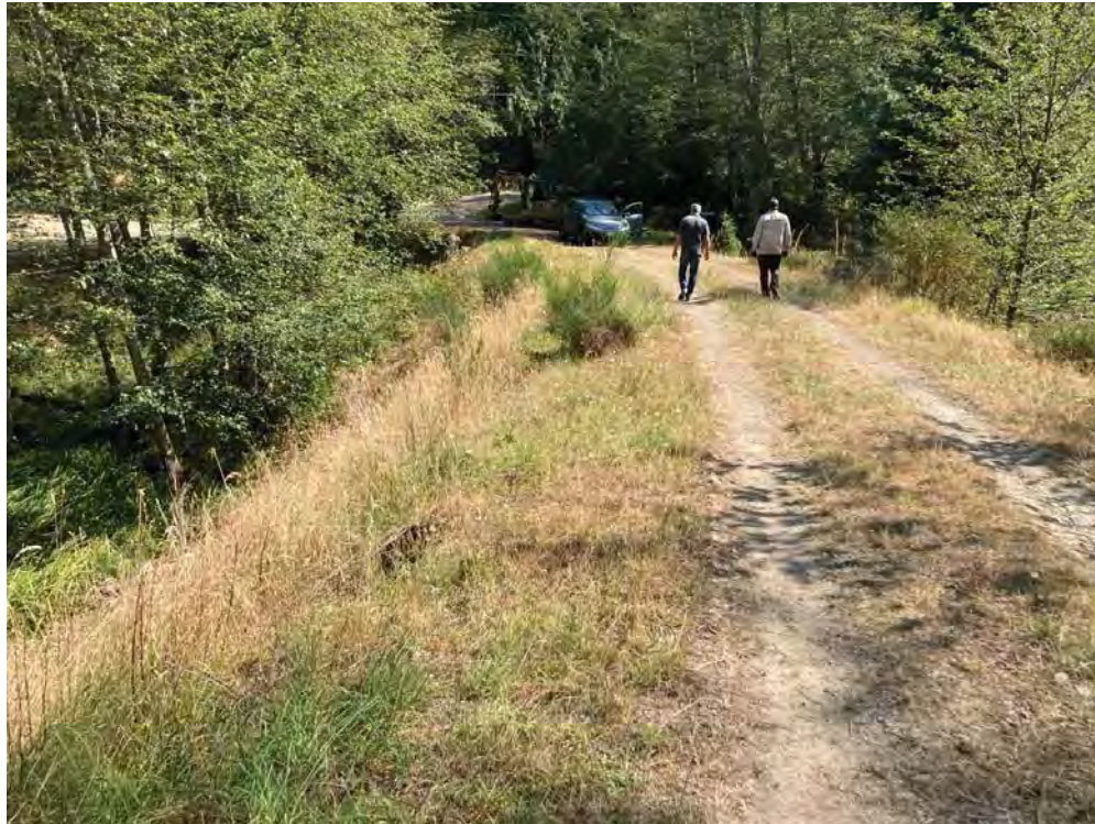
Photo 23: Money Diversion Dam located ~450 m downstream of Money Dam No. 1. (2022-08-31, JDM)
