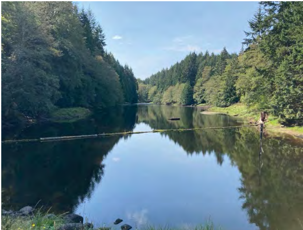
Photo 2: Looking some at reservoir from dam crest. (2022-08-31, JDM)
