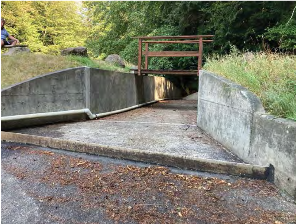
Photo 7: Looking north at entrance to spillway. Note seepage return pipe. (2022-08-31, JDM)
