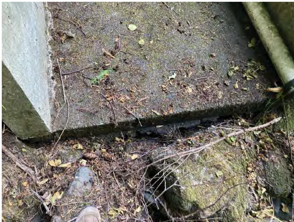
Photo 10: Downstream of spillway chute. (2022-08-31, JDM).
