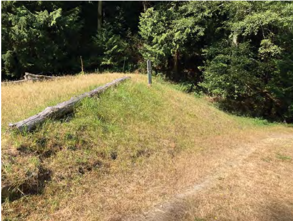
Photo 13: Downstream slope. (2022-08-31, JDM)
