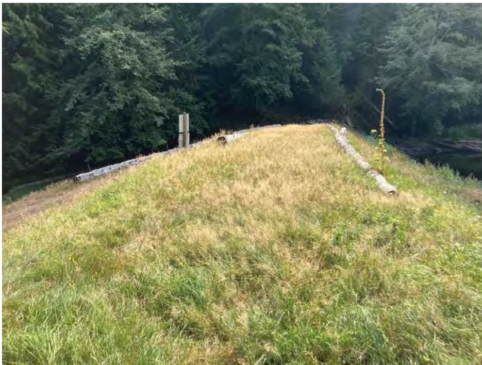
Photo 12: Dam crest from left abutment. (2022-08-31, EPS).
