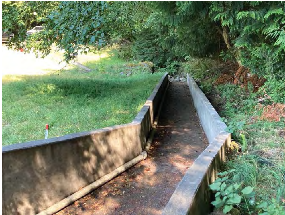
Photo 9: Spillway chute at right abutment (2022-08-31, JDM).
