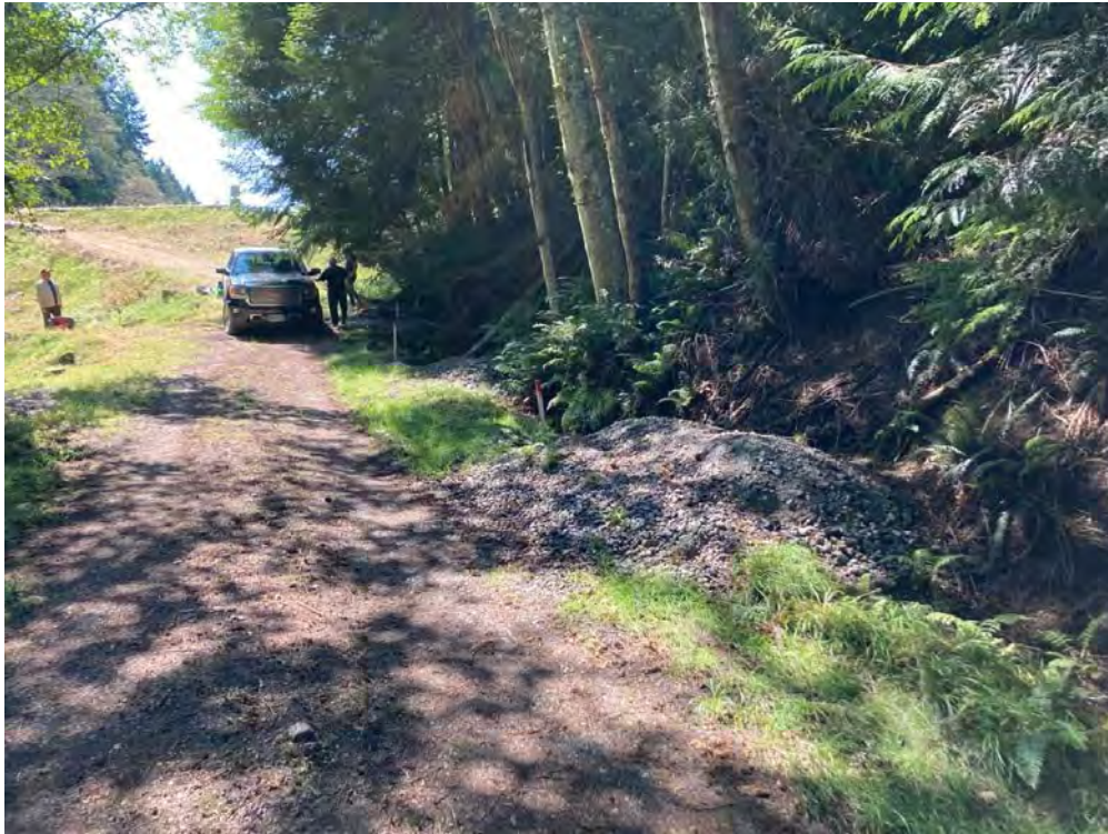
Photo 21: Seepage collecting infrastructure downstream of left abutment. (2022-08-31, JDM)
