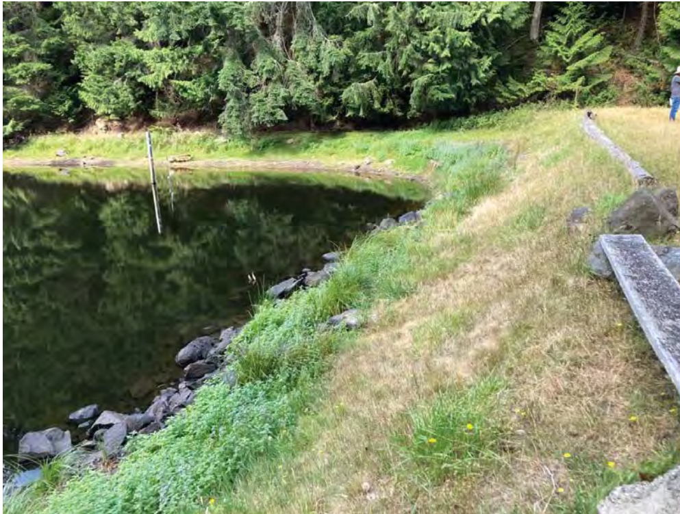
Photo 11: Upstream slope of dam from right abutment. (2022-08-31, JDM)
