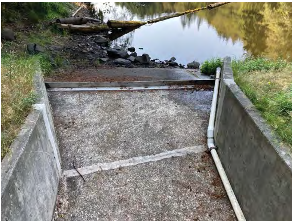
Photo 8: Spillway entrance. Note aluminum weir plate. (2022-08-31, JDM).
