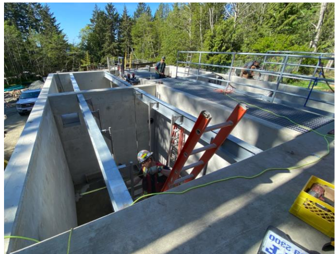
MBR Tanks – Structural Steel
