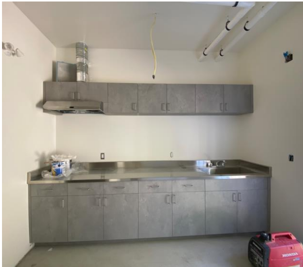
Lab and Control Room
