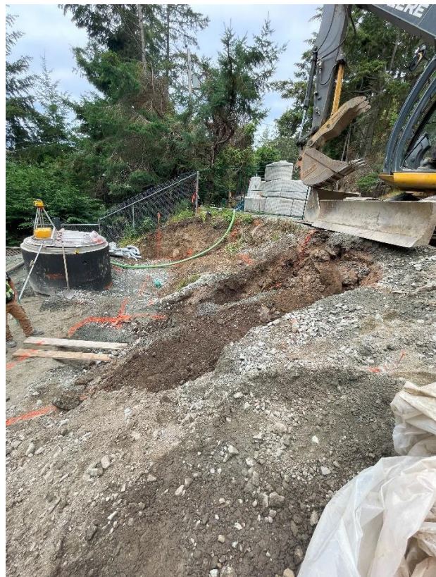
Cannon PS – Prep for Lockblock Wall
