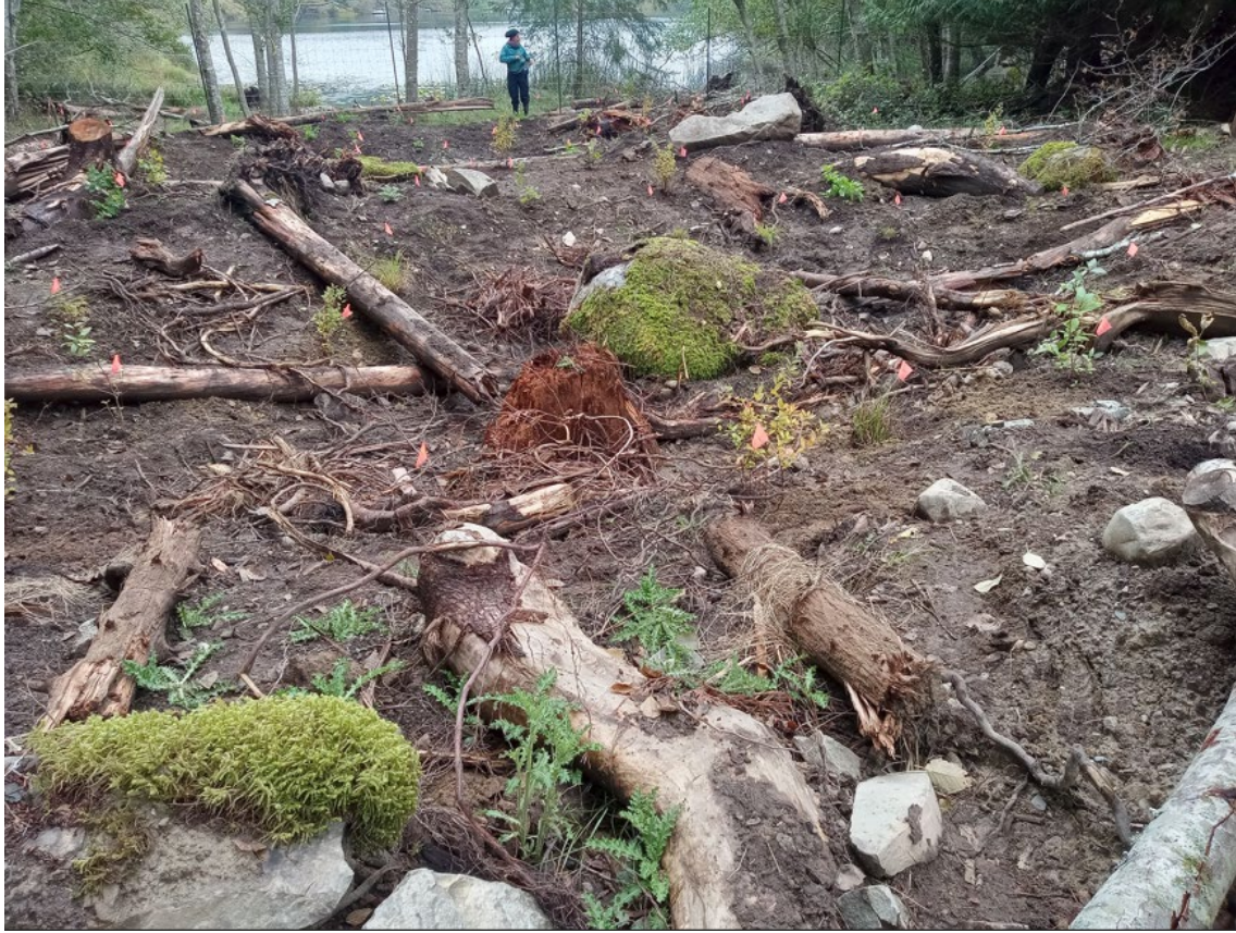
Wetland Restoration beside Galleon PS and Buck Lake
