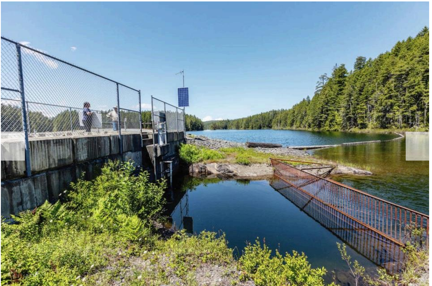
1 / 8 The crown jewels of the catchment area for the Capital Regional District's Regional Water Supply Service are the five stream-fed reservoirs — including the largest, Sooke Lake — that collectively hold 170-million cubic metres of water. DARREN STONE, TIMES COLONIST
