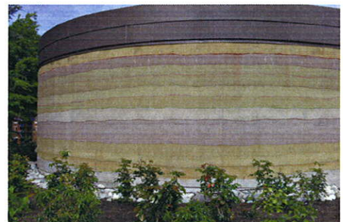
Rammed earth building, Saanich, BC
