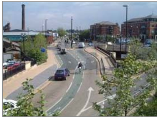
Figure 2. Separated Bicycle Lanes at a Transit Station in the City of York, UK
