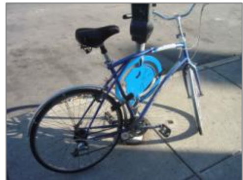
Figure 1. Stationnement de Montreal parking meter retrofit for short term bicycle parking.
